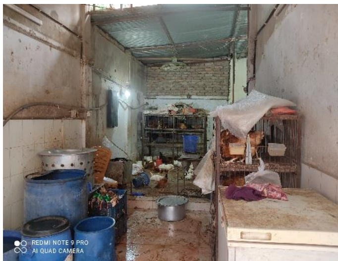
Fig. 3: Existing condition of the selected single-shop LBM
