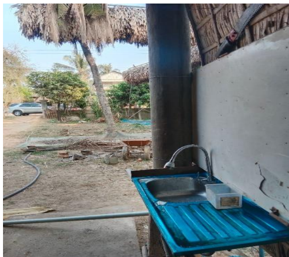
Figure 4. A new handwashing facility installed by a BGP in Varint 3 village.
